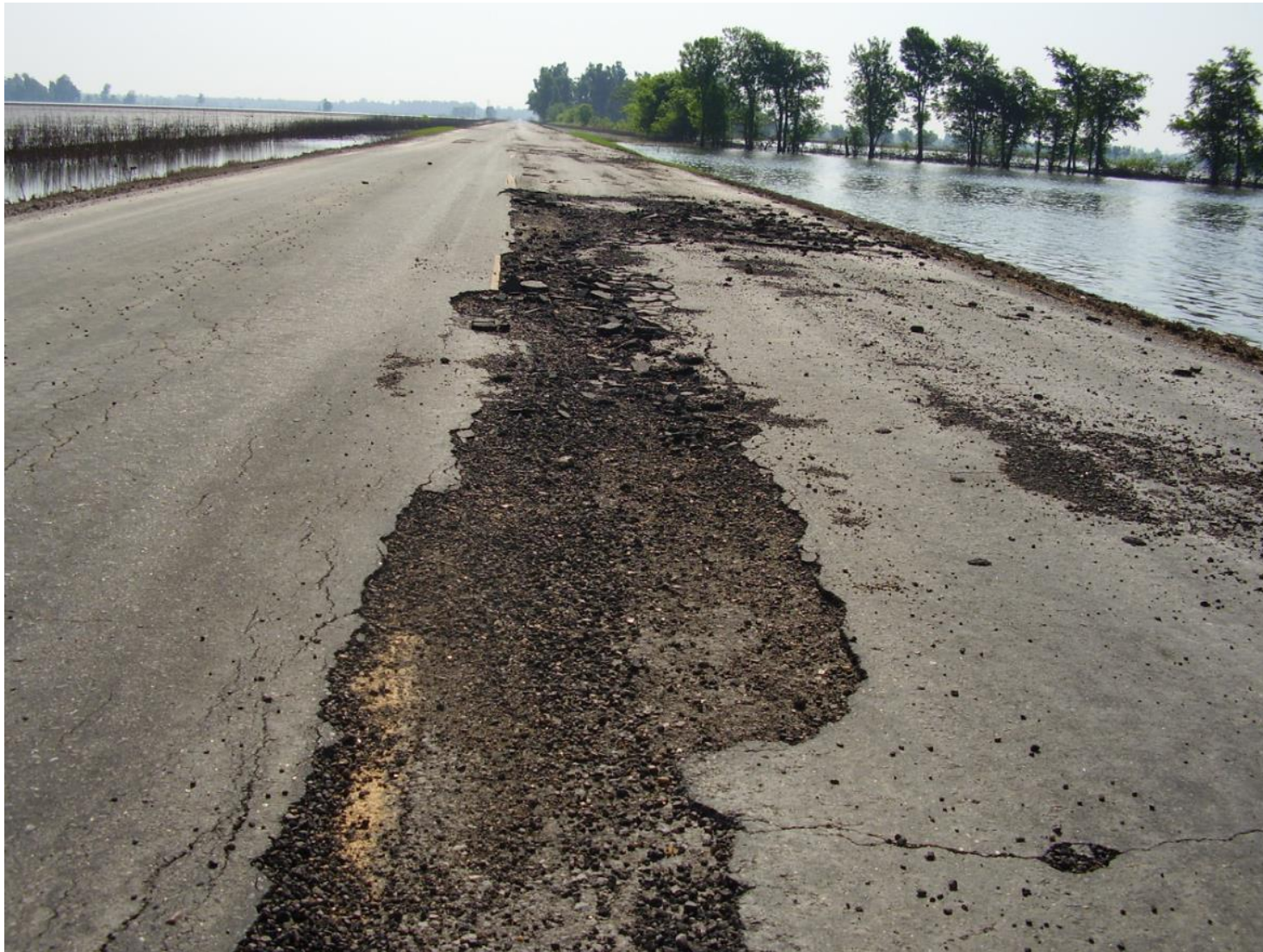
Heavy Delamination
